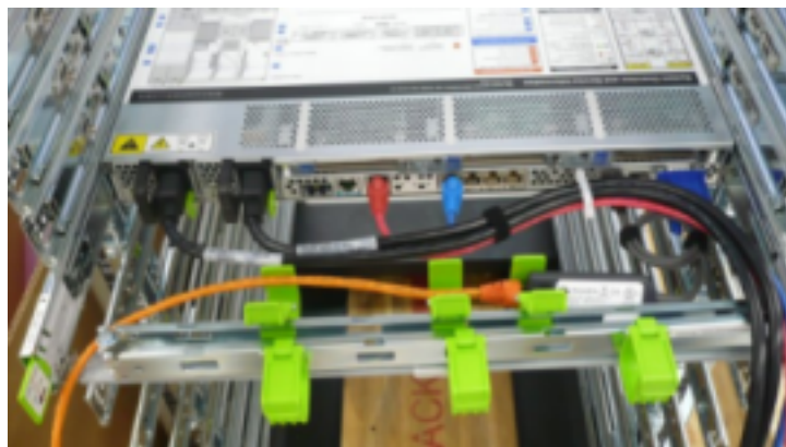
Figure 2-5 Cables Routed Through the Cable Management Arm
